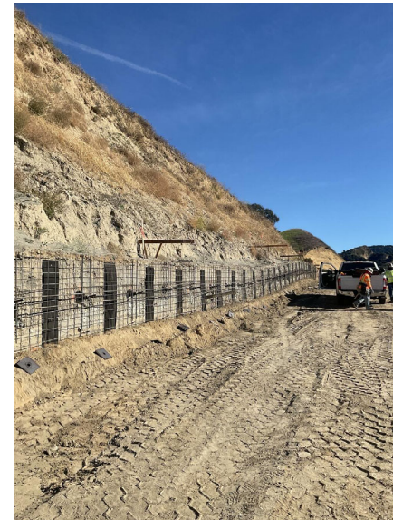
Soil nail installation at Retaining Wall 2524
