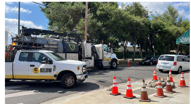
Sidewalk Panel Restoration on Bessemer St
