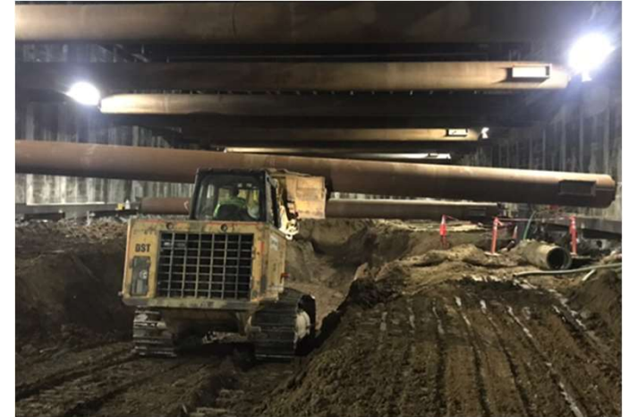
Westwood/UCLA Station: Placement of BL3 Strut
