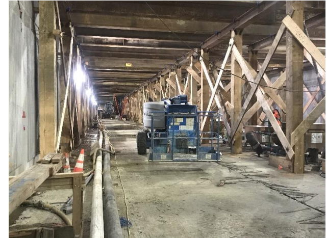
Century City Constellation Station Falsework for 2 nd level wall construction at east end
