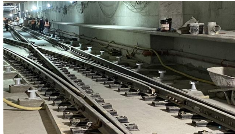
Wilshire/La Cienega Crossover Track Third Rail Pedestal Installation
