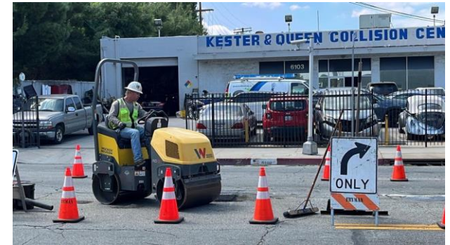
Potholing Restoration on Bessemer St.
