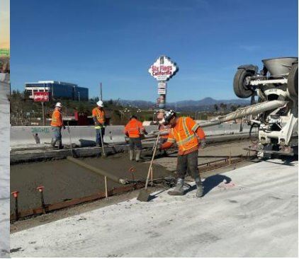
Placement of Lean Concrete Base (LCB) in the median
