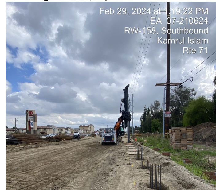
SR-71 SB, SW158 CIDH pile construction.
