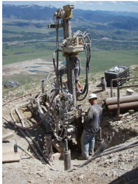
Image 15 – Example of low-impact micropile foundation construction.
