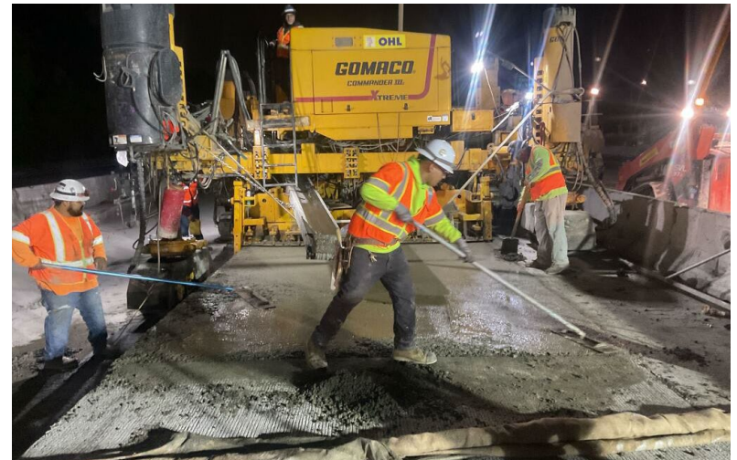
Jointed Plain Concrete Paving in Median
