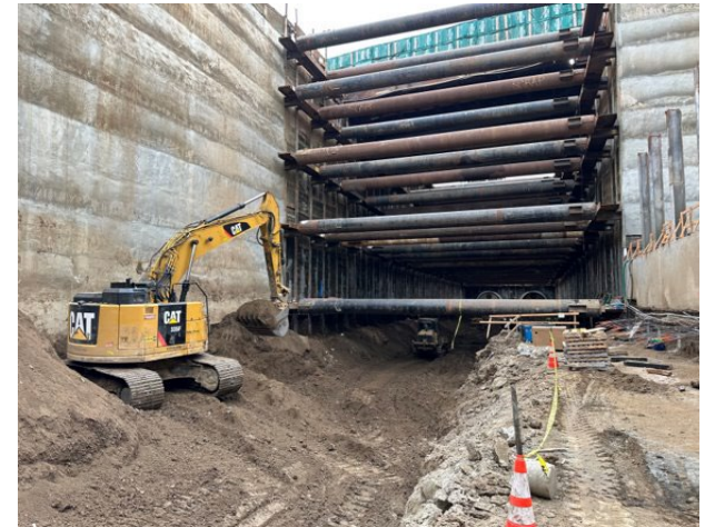
Westwood/VA Hospital Station: Excavation in Station Box
