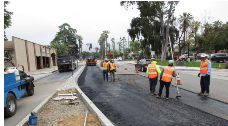
San Dimas Avenue – Roadway Paving
