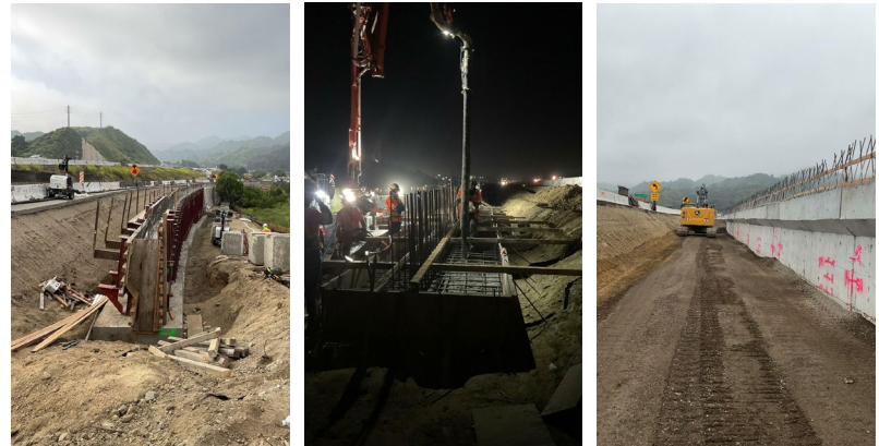
On-going work at Retaining Wall 2577
