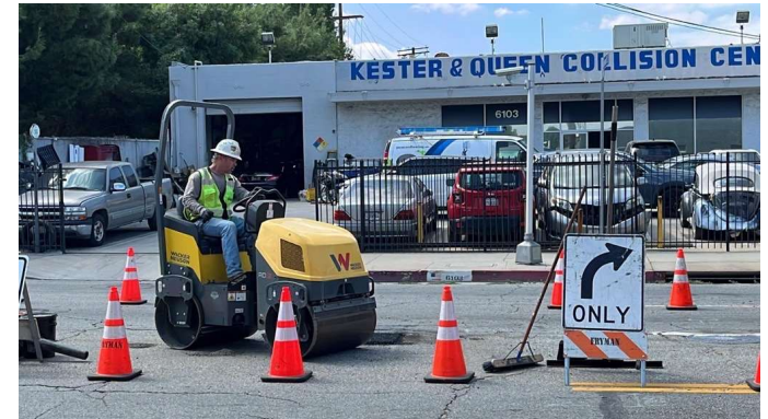
Potholing Restoration on Bessemer St.
