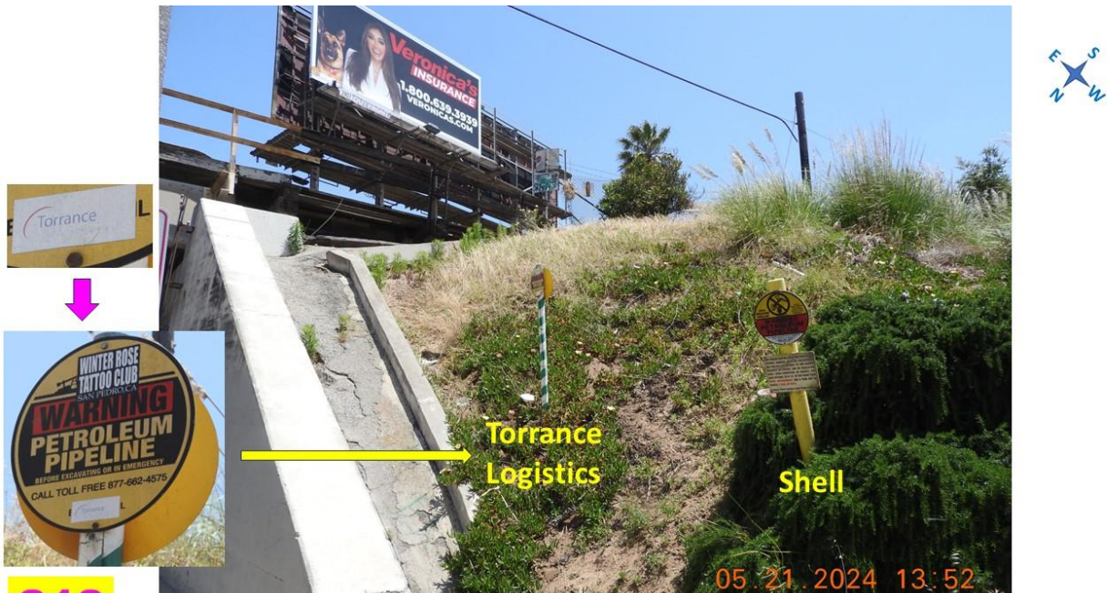
S12 Looking southeast at Southwest corner of Artesia and Freight Track Bridge
