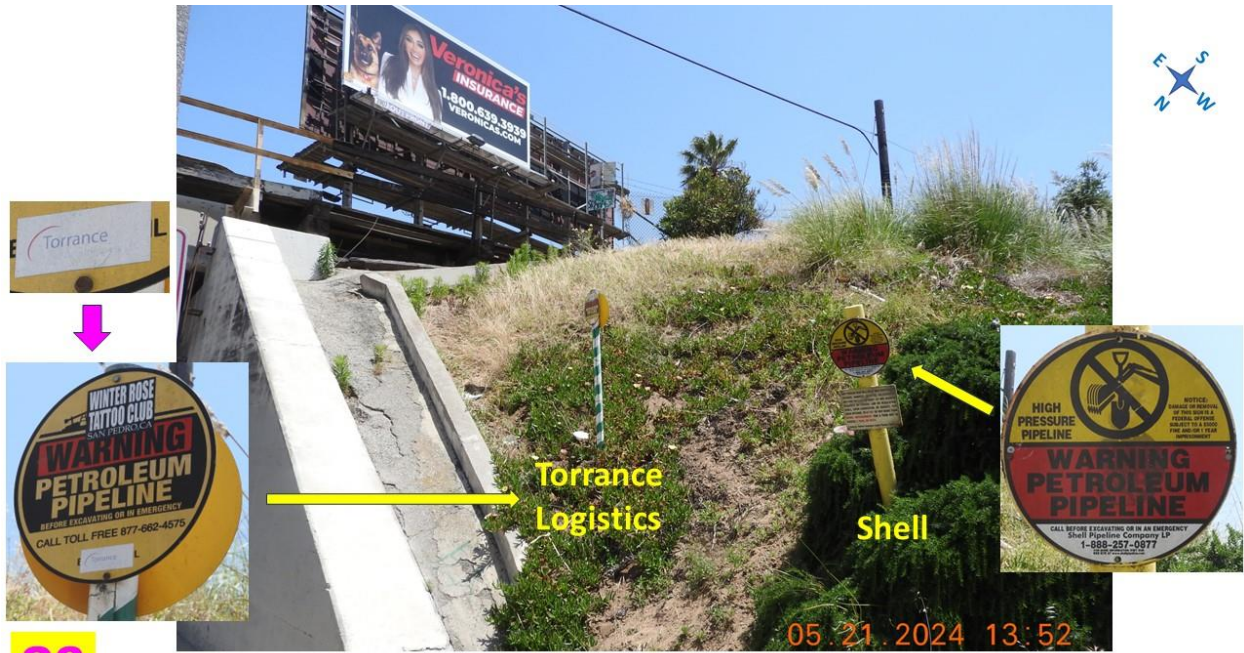
S3 Looking southeast at Southwest corner of Artesia and Freight Track Bridge
