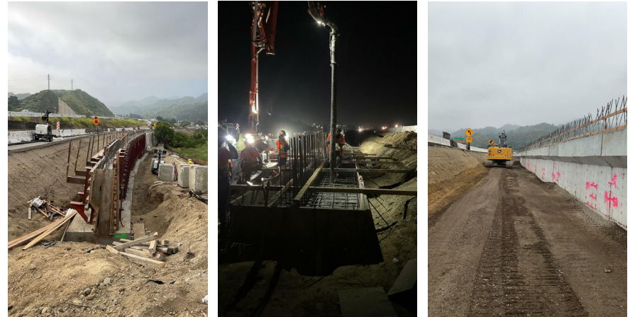
On-going work at Retaining Wall 2577
