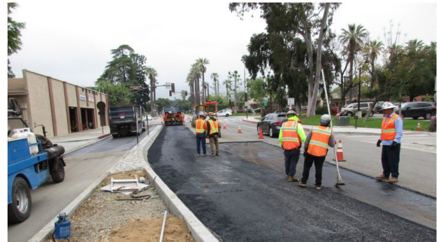
San Dimas Avenue – Roadway Paving
