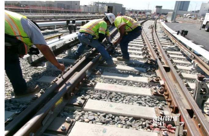
QC Track Inspection
