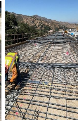
Gavin Canyon Bridge Deck Rebar Install
