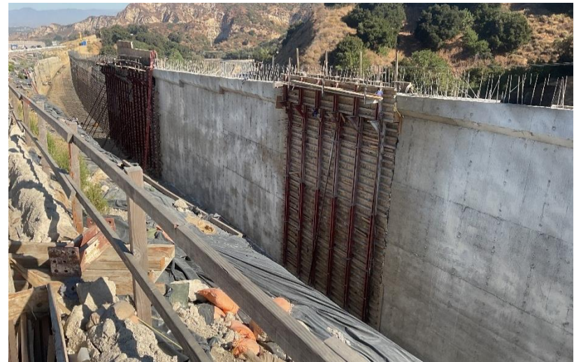
Retaining Wall 2460 formwork installation
