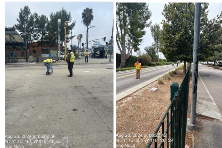
Phase II Environmental Site Assessment – Site Walk & Soil Boring Marking at Van Nuys
