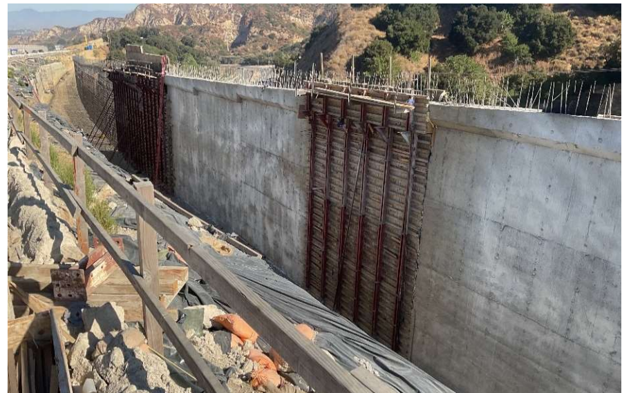
Retaining Wall 2460 formwork installation
