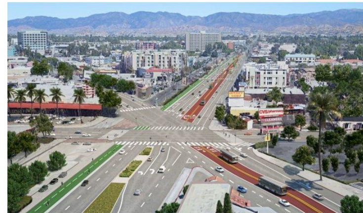
View of Vineland Ave / Lankershim Blvd
