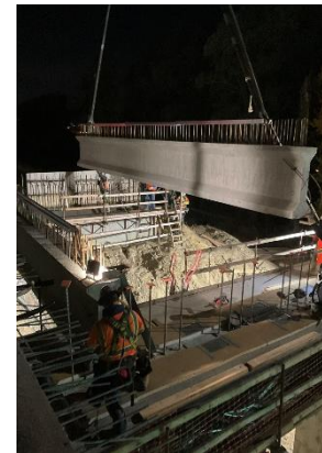
Set Girders at Rye Canyon Bridge
