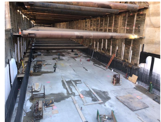
Westwood/VA Hospital Station: Completed Invert Concrete Pours (Looking West)
