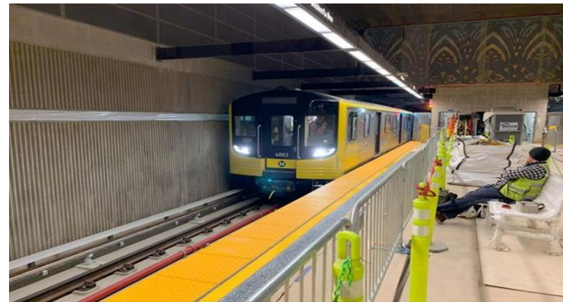
Reach 1 Tunnel (Western to La Brea) Live Car Train Test entering Wilshire/La Brea Station
