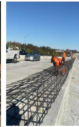
Median Barrier Rebar Installation
