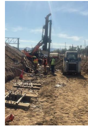
Wall 986 Installation of 24IN CIDH Piling
