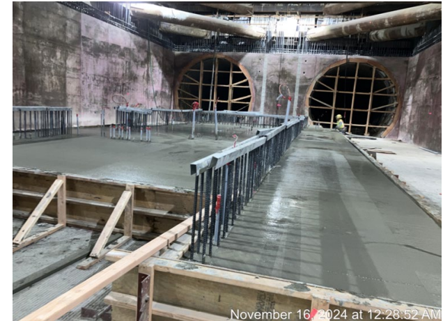
Westwood/UCLA Station: Secondary Invert Concrete Pour (East End)
