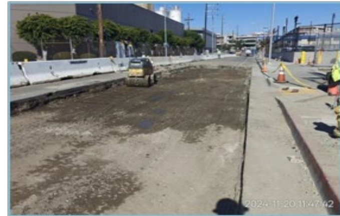
Center Street Reconstruction
