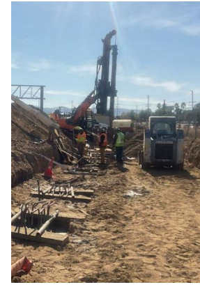
Wall 986 Installation of 24IN CIDH Piling
