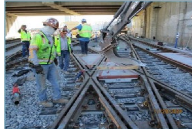
Crossing Panel Installation
