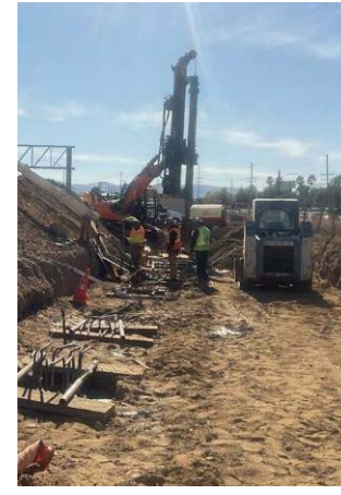
Wall 986 Installation of 24IN CIDH Piling
