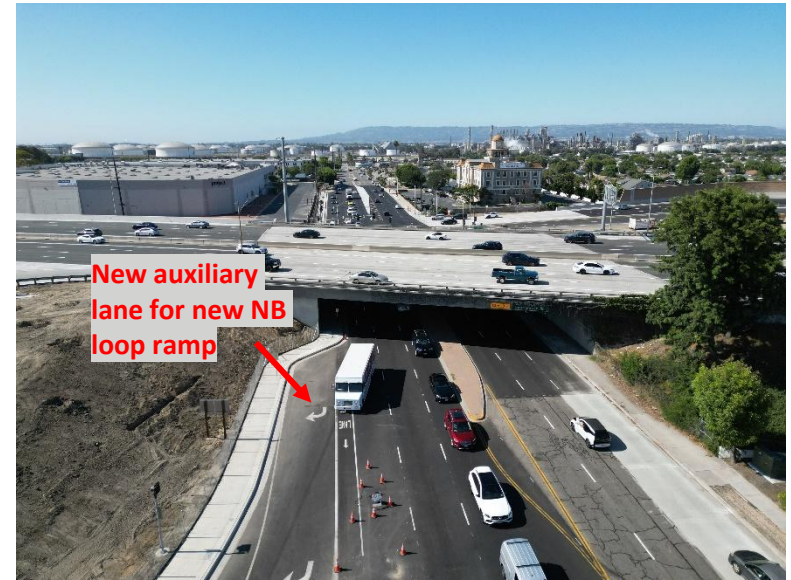
North side of Crenshaw Blvd UC (Looking South) showing Crenshaw Blvd improvements/auxiliary lane for new NB loop ramp.
