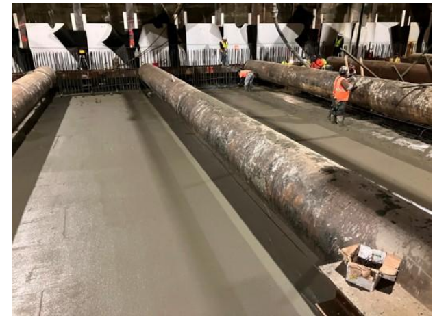
Westwood/VA Hospital Station: Concourse Deck Slab Concrete Placement (Looking South)
