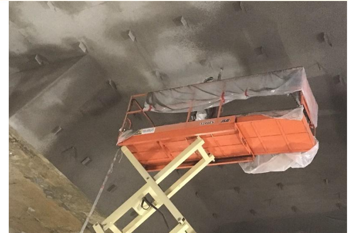
Century City Station Acoustical Treatment on Ceiling
