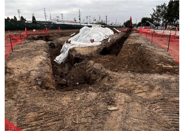
Storm Drain Removal at Van Nuys
