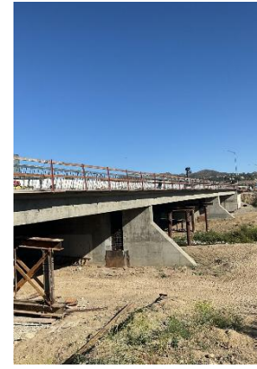
Castaic Creek Bridge Falsework Lowering
