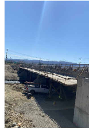
Rolled Soffit at Castaic Creek Bridge NB I-5
