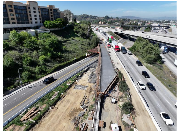
Golden Springs Drive Undercrossing Bridge Deck Placement.
