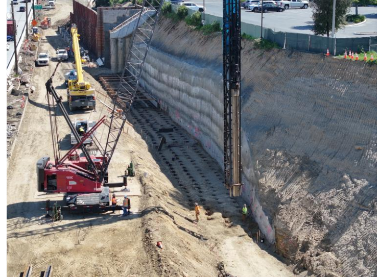
Driven piles for northbound SR-57 Retaining Walls.
