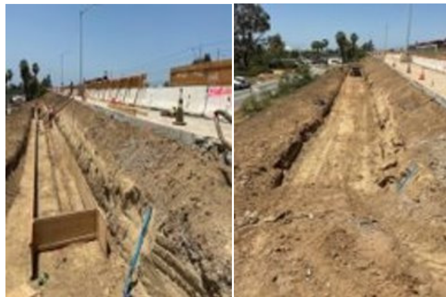
RW 245 Forming Footing
