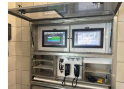
Wilshire/La Brea Station: Testing Emergency Management Panel
