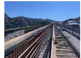
Gavin Canyon Bridge Right Formwork
