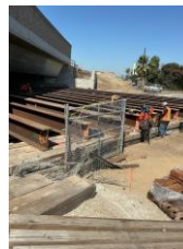
105WB-Dominguez Channel - Setting falsework beams
