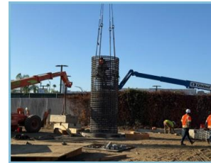
Setting Column Cage at Van Nuys Bent 25
