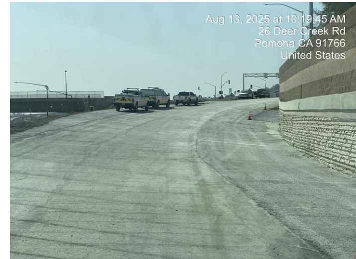
Realigned SB Rio Rancho off-ramp, LCB paving.
