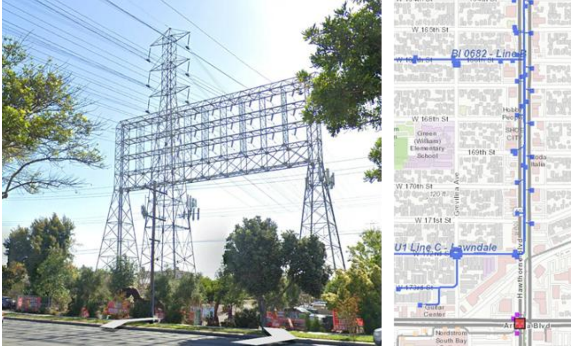
Photo of utility corridor with high voltage transmission lines that cross Hawthorne Blvd (Google street view) and diagram of major storm drain located in center of Hawthorne Blvd, to be relocated for Hawthorne Blvd Option (Metro, 2025)
