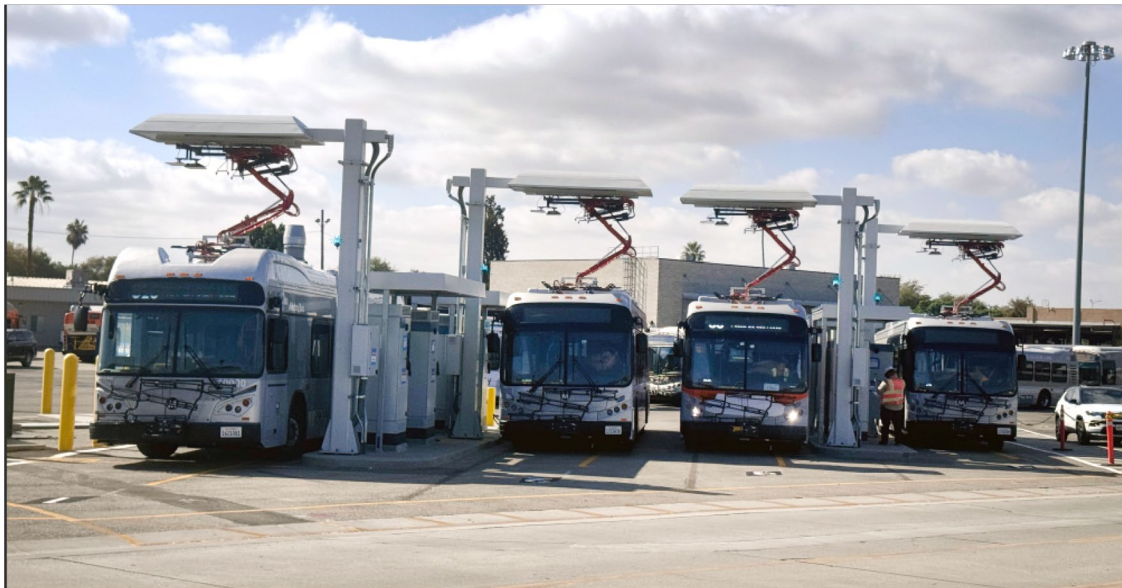
Photo: Division 9 Bus Yard Opportunity Chargers
