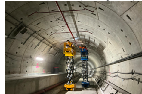
Tunnels: Tunnel Lighting Installation Reach 7 BR Tunnel
