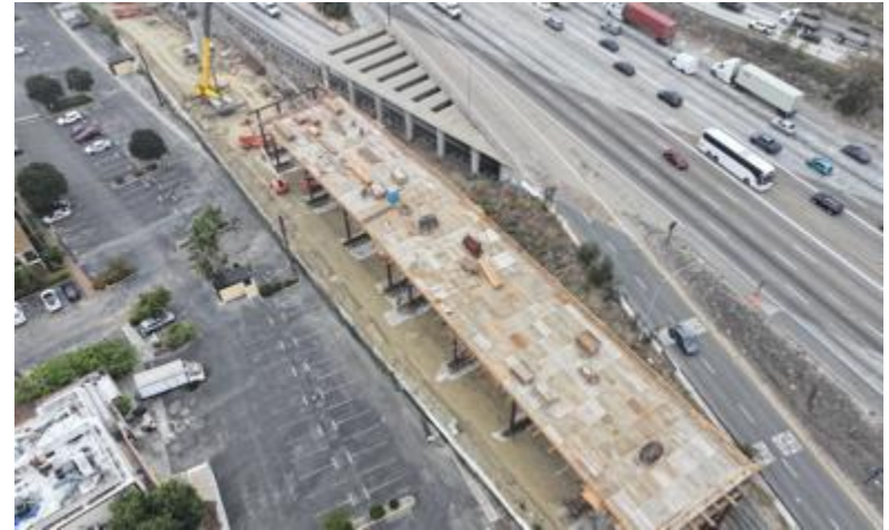
Falsework for EB SR-60 Bypass Bridge Deck
