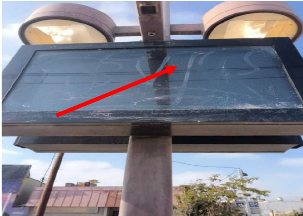
Pico/Aliso Station: 2024E-001 July 29, 2025 - Broken Monitor
