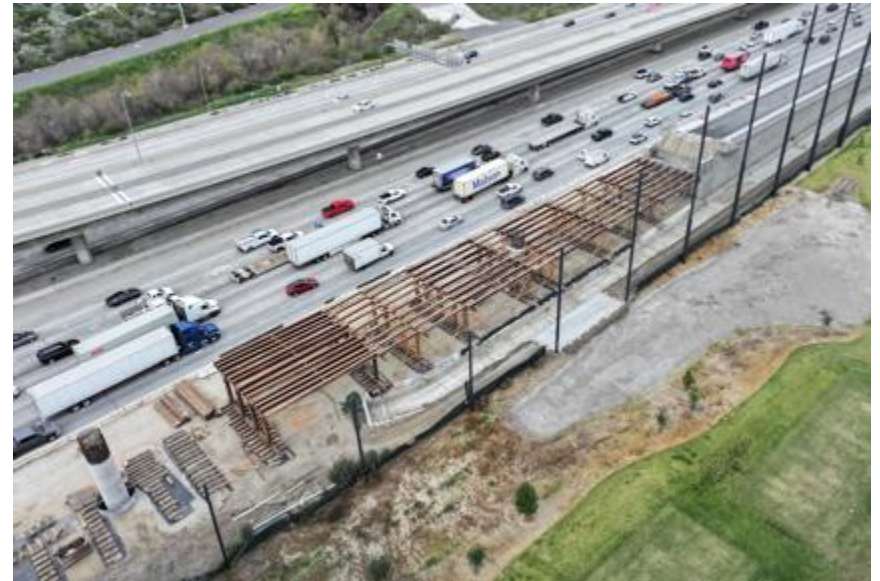
Erection of falsework for EB60-Grand Ave/N57 Separation
