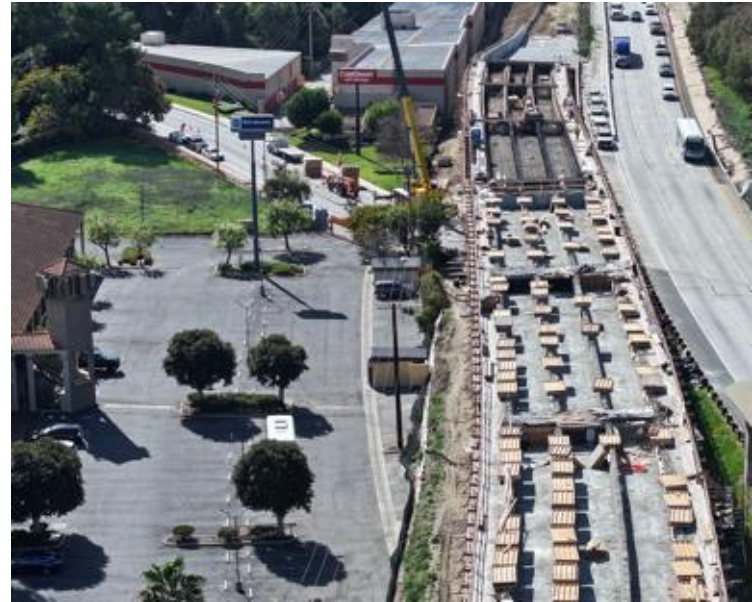
Placement of rebar and formwork for EB SR-60 Bypass bridge
