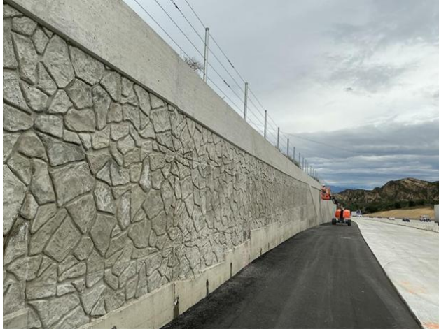
Roadway Excavation Southbound Hasley to Parker
