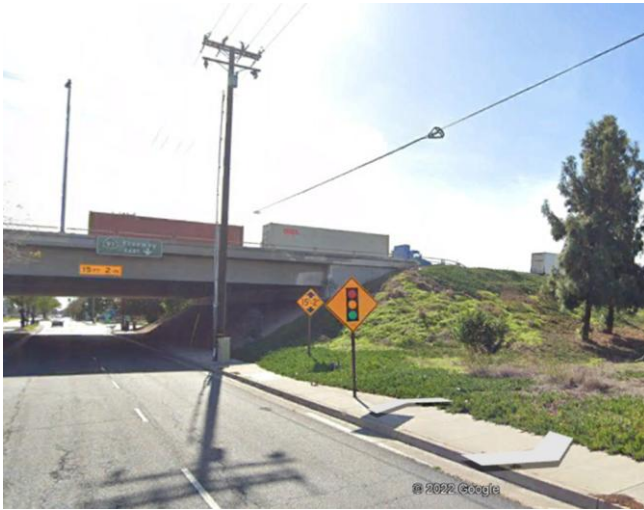
Utilities Relocation at Norwalk Blvd. (North SR-91)
