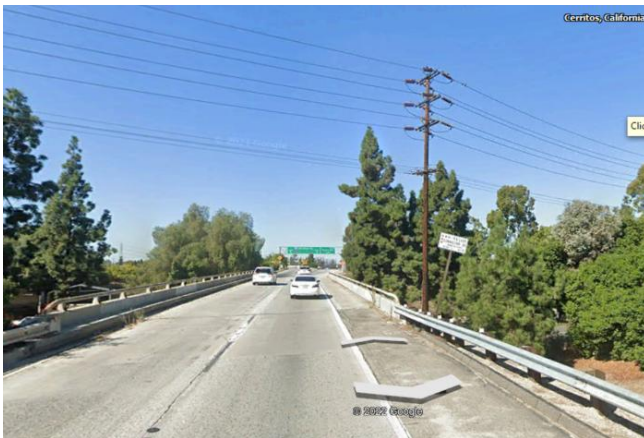
WB 91 to 605 Connector - Utilities Relocation at Studebaker
