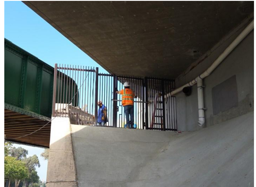
Reinforced security gate installation - Route 66 under bridge area
