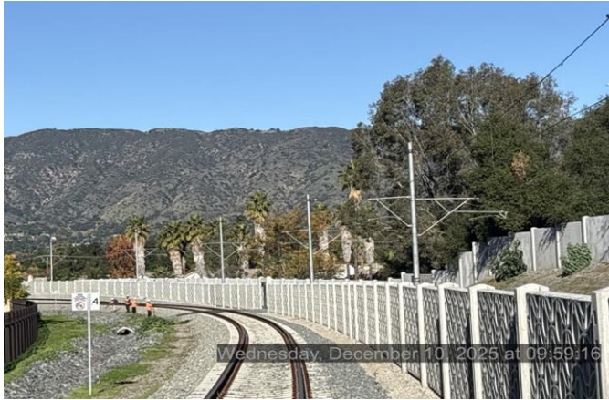
Weed abatement along the LRT corridor - Loraine to Lone Hill
