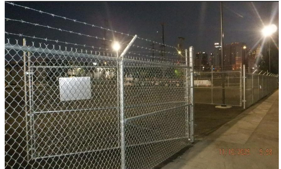
Fencing & site lighting installed (December 2025)
