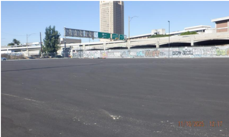
Building demolition & site paving complete (December 2025)
