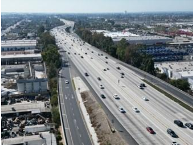
EB Cherry Ave Off Ramp
