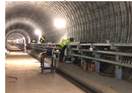
Tunnels: Steel Walkway Construction BL Tunnel
