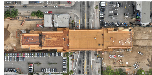
Aerial View of Van Nuys Bridge Construction
