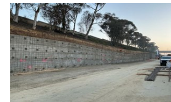
105WB RW 270 Soil Nail Wall Exterior
