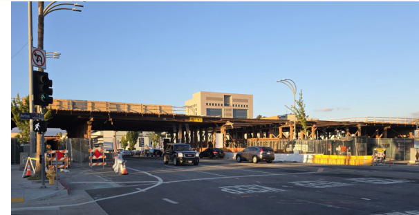
Falsework for Van Nuys Bridge
