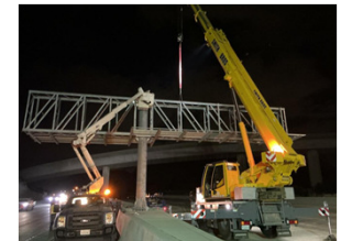
Sign Structure Truss Installation
