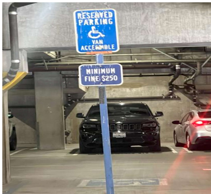
Picture 14 3/11/2026 - Union Station Worn Out Sign/Some Deterioration
