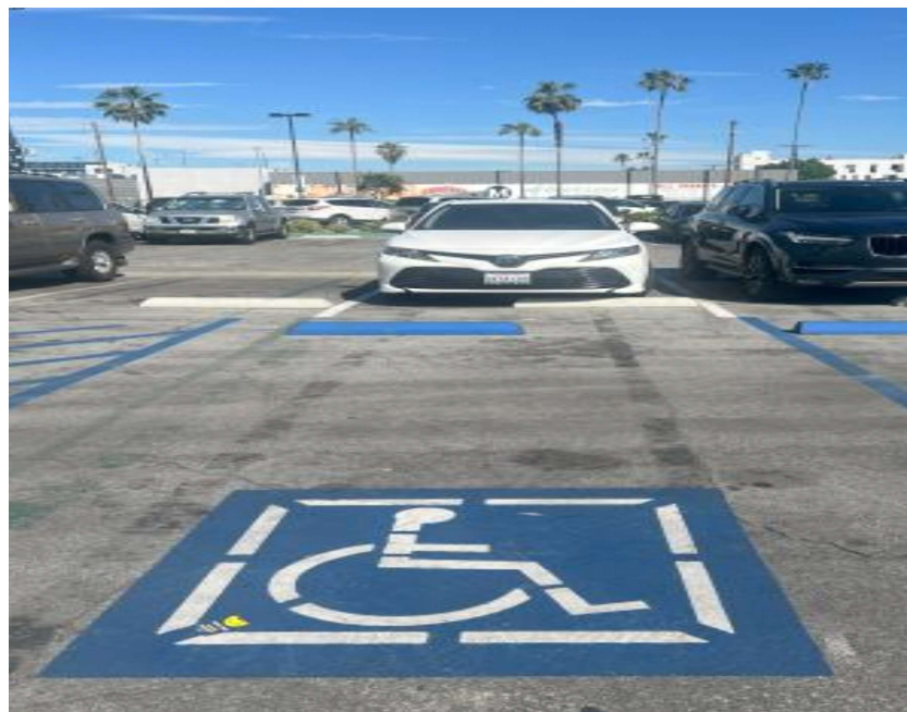
Picture 12 2/26/2026 – North Hollywood (B Line) No Vertical ADA Sign
