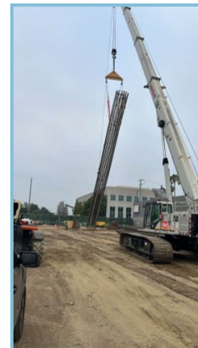
Setting Cages for CIDH Piles at Sepulveda
