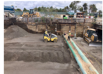
Westwood/VA Hospital Station: Main Box Backfill Operation
