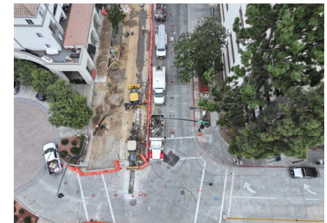
Holly and Arroyo Westbound Station Construction
