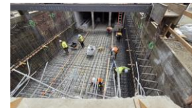
Pacoima Wash Box Culvert Replacement
