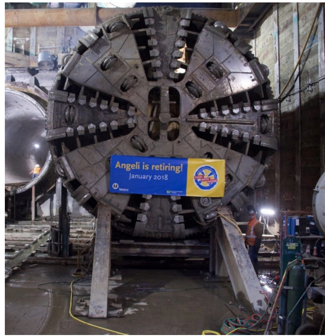
Tunneling completed January 16, 2018
