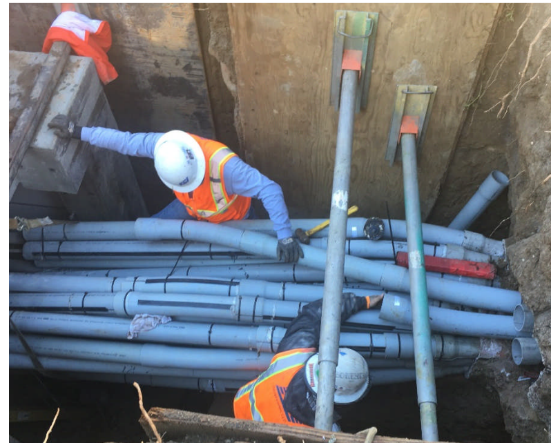
AT&T Conduit Installation in Century City
