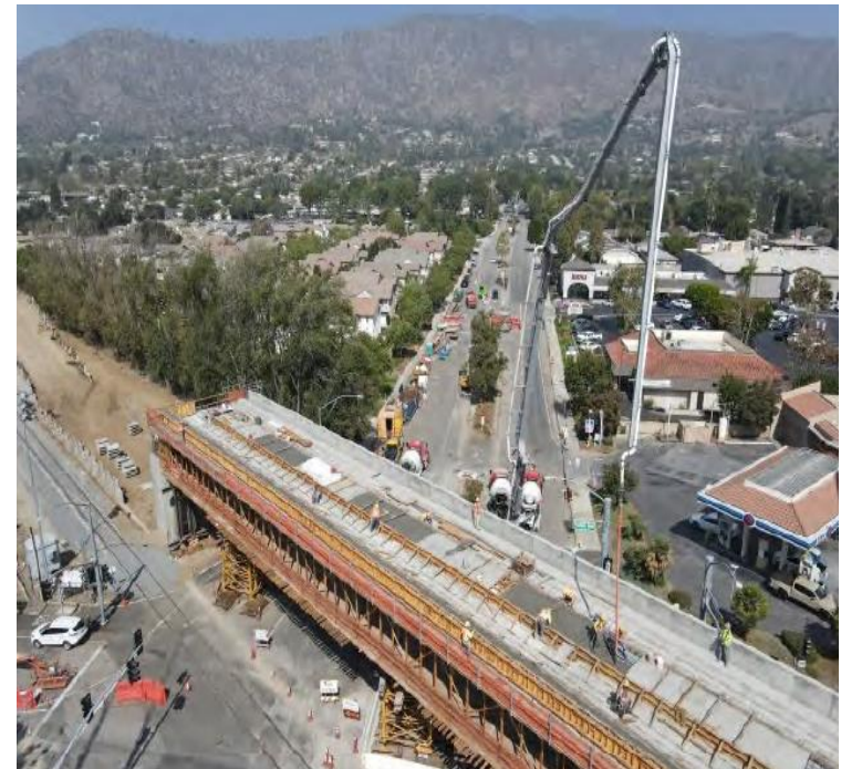
Foothill Grand - LRT ductbank walkway
