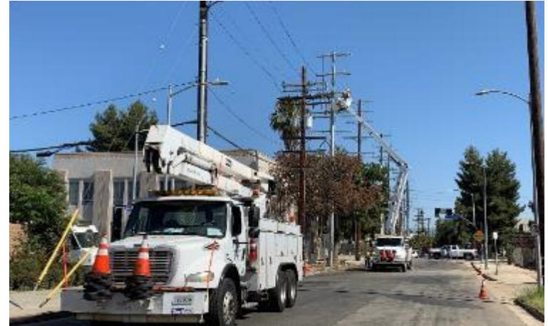
DWP Overhead Construction at Vesper
