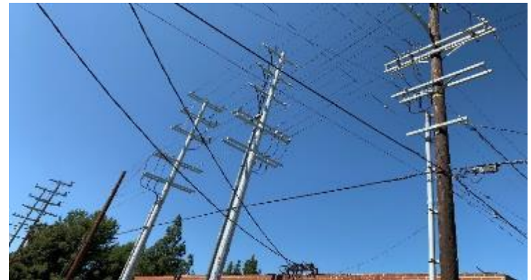
DWP Overhead Construction at Vesper
