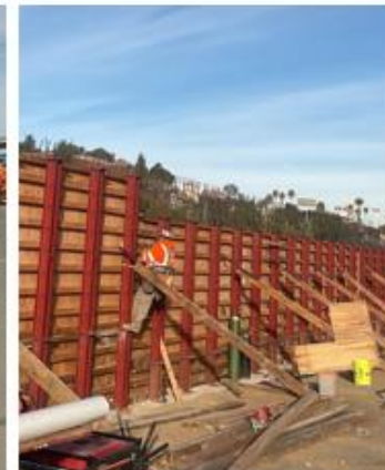
Forming, preparations, and concrete pour at Retaining Wall 2622
