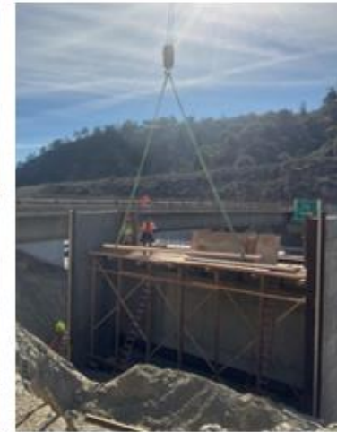
On-going abutment and wing wall construction at new Weldon Canyon Bridge
