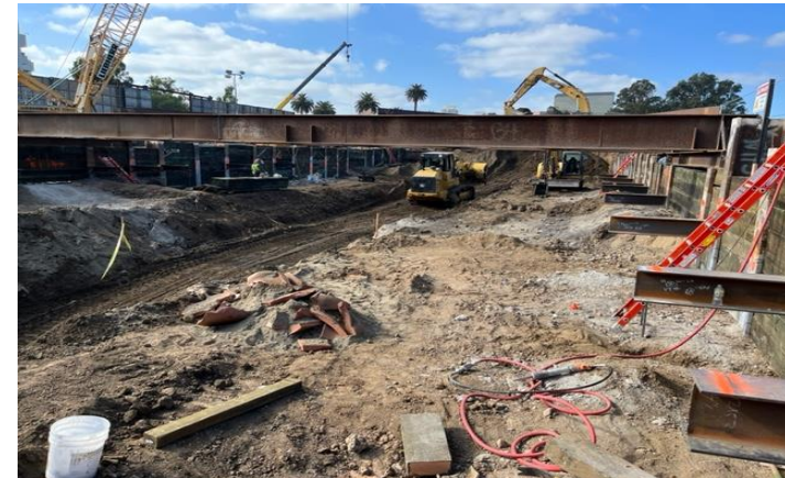
Westwood/VA Station: Excavating station to Level 1 Bracing
