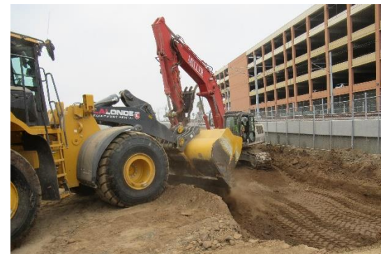
On Site Backfilling Work
