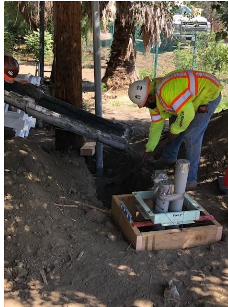
Pilot Gate - DWP Service Pedestal Installation
