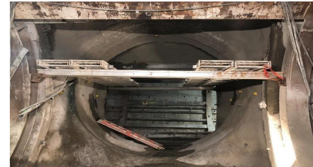
Excavation Complete at Cross Passage #16 (Reach 2)
