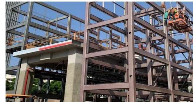
Welding for elevator hoist way frames at Grand Av Arts/Bunker Hill Station
