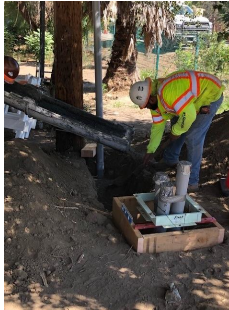
Pilot Gate - DWP Service Pedestal Installation
