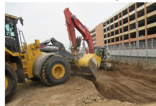
On Site Backfilling Work
