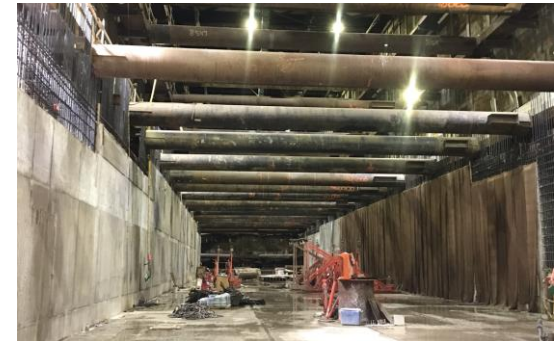
First Level Walls at Wilshire/Rodeo Station
