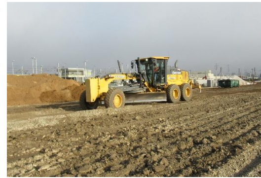
Backfill Work at South End of Site
