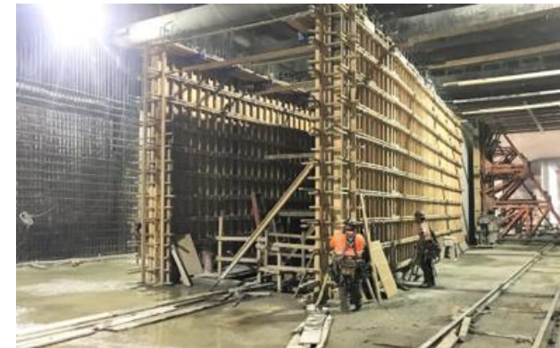
East Interior Wall Formwork at Wilshire/La Cienega
