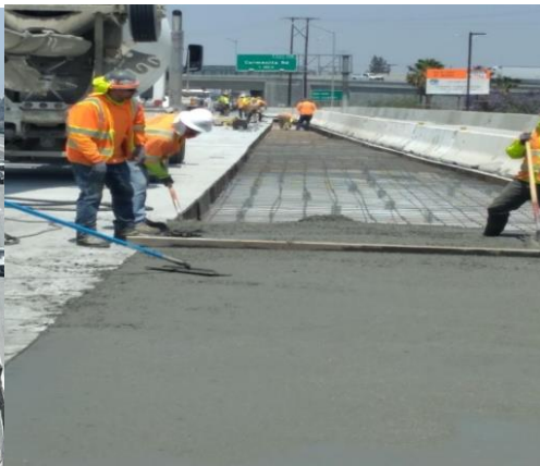
Paving Operations on NB freeway lanes
