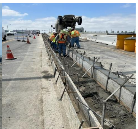
Valley View median construction
