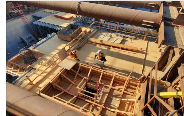
Wilshire/Fairfax Entrance Roof Construction
