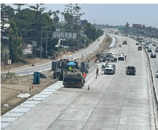
Paving along NB freeway lanes
