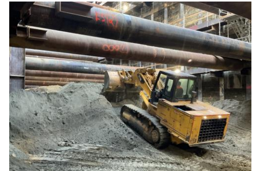
Constellation Station Excavation Activities
