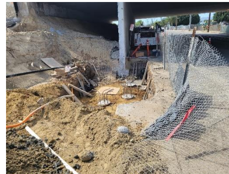
NE side of Van Ness Ave Bridge Widening showing CIDH for footing – looking South
