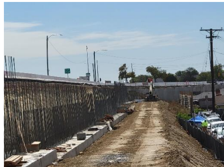
RW 815 and RW 808 – SB 405 Crenshaw Blvd off ramp widening – Looking South
