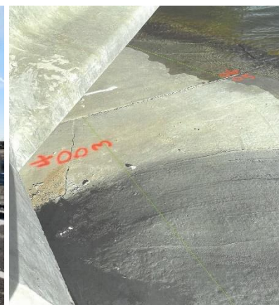
Channel Lining Cracks
