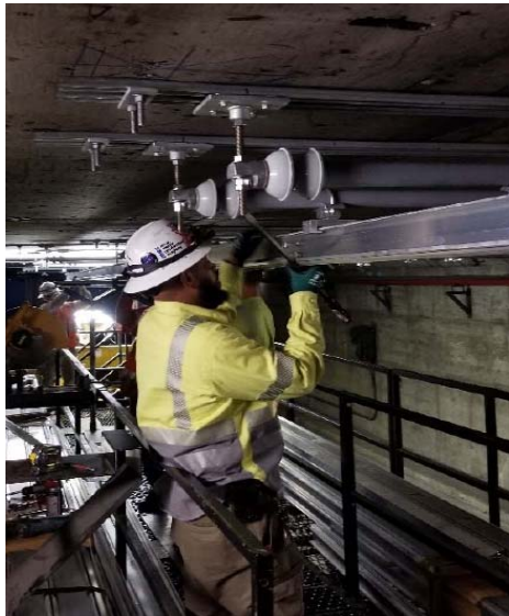
7 th Metro tail track new Overhead Conductor Rail (OCR)
