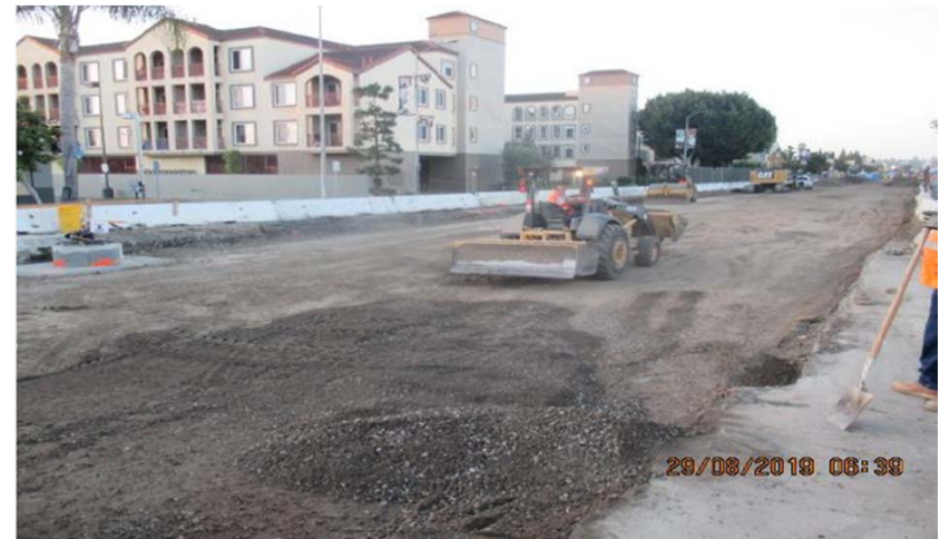
Continued restoration 60th to 63 rd Streets at UG#3
