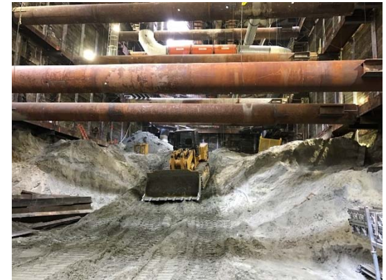
TBM Launch Box Excavation in Century City
