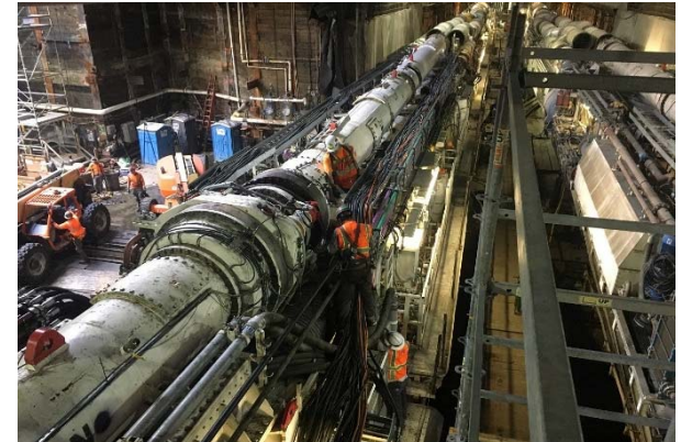
TBM Assembly at Wilshire/La Brea Station
