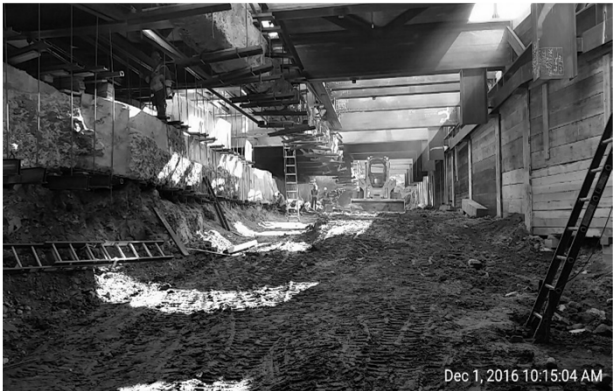
Utility hanging within 2 nd /Broadway excavation
