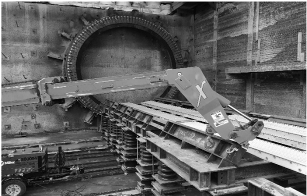
Thrust frame assembly and eye seal
