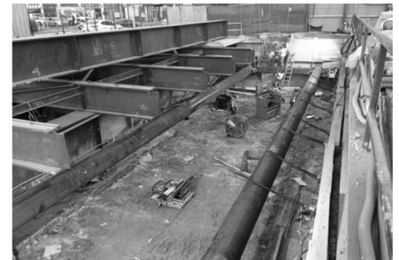
Installing Strut at Wilshire/La Brea Station
