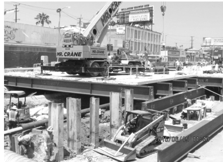
Vernon Station Decking
