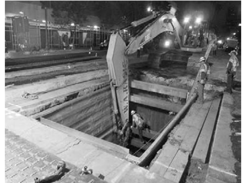
Setting Power Vault on Wilshire
