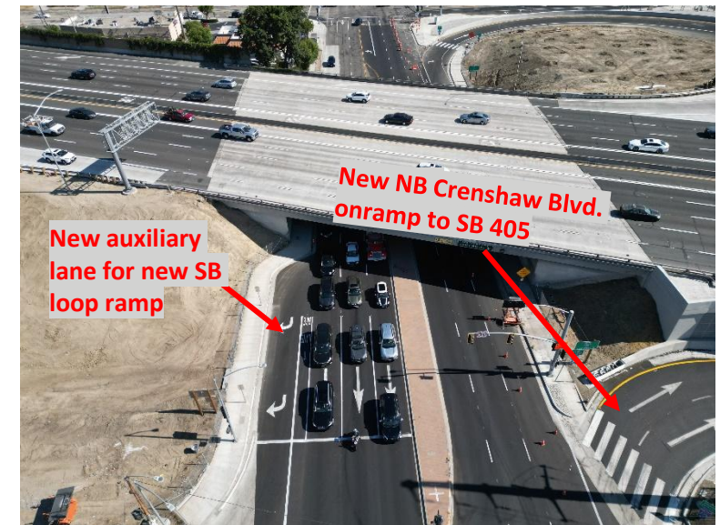
South side of Crenshaw Blvd UC (Looking North) showing Crenshaw Blvd improvements/auxiliary lane for realigned SB on ramp and new NB Crenshaw Blvd to SB 405 on ramp
