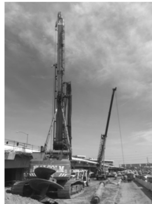
First pile drilling
