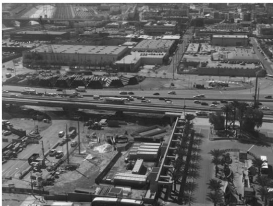
Aerial view of site
