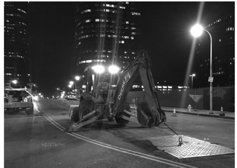
Telecom Joint Trench Construction along Constellation Boulevard
