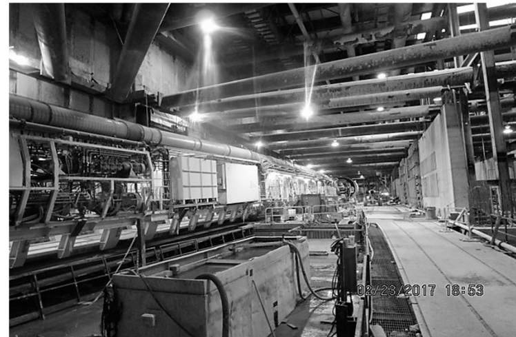
TBM trailing gear being pulled thru MLK Jr. Station
