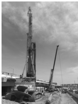
First pile drilling
