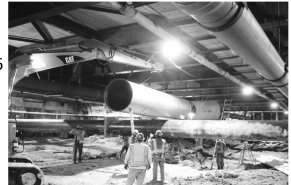
Pipe Strut at Wilshire/La Brea Station
