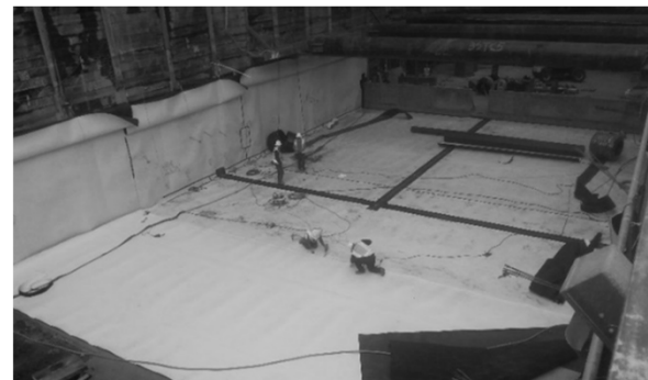
HDPE placement at 2 nd /Hope Station
