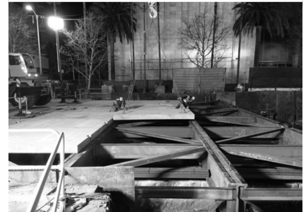
Placement of Deck Panel at Wilshire/Fairfax
