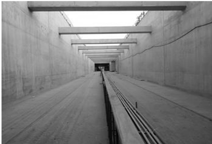
Completed wall sections of Tunnel near airport runways
