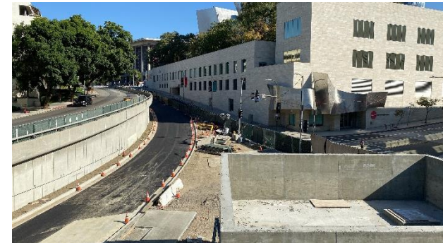
Concrete curb & gutter at 2nd Place/Flower
