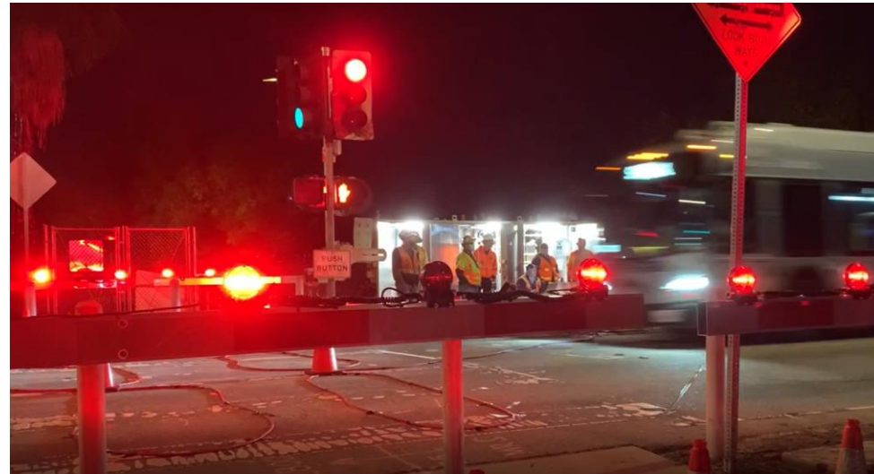
Pilot Gate - Testing
