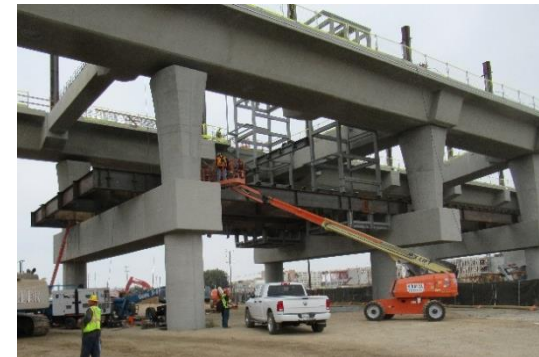
LAWA APM Steel Work in Progress
