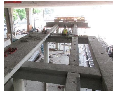
Precast @ Blue Line Mezzanine Extension
