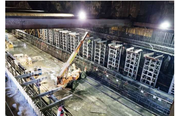
Wilshire/Fairfax Station Concourse Shoring
