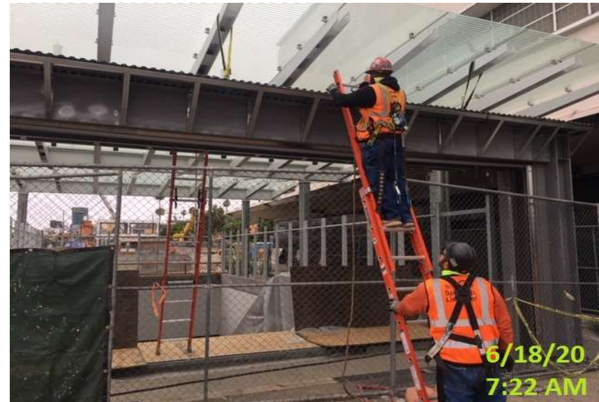
Installing roofing deck to main entrance canopy at MLK Jr. Station.
