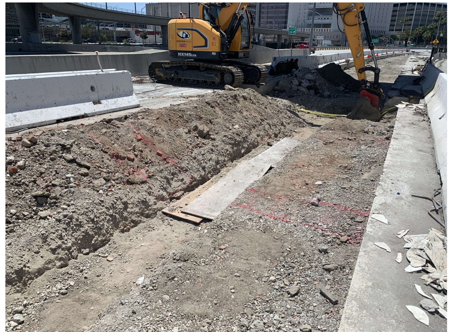
Archaeological Data Recovery Begins at Storm Drain
