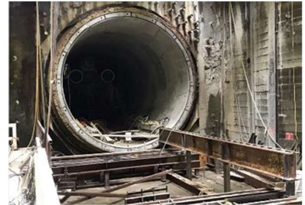
BL Tunnel at the Launch Box in Century City
