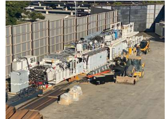
TBM Components at VA Staging Yard
