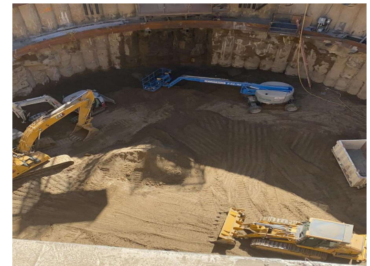
TBM Launch Shaft Excavation
