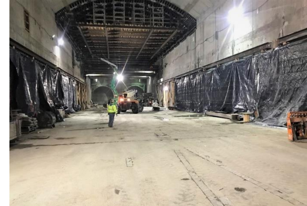
Track Level View of Wilshire/La Cienega Station
