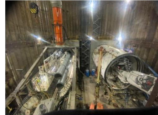
TBM Assembly Overview at Tail Track Exit Shaft
