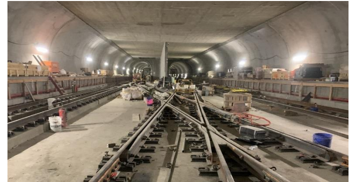
Special trackwork installation in Crossover Cavern
