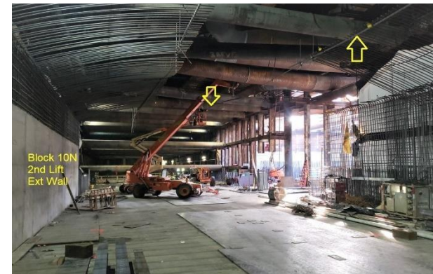
Installing Roof Rebar at Wilshire/Fairfax
