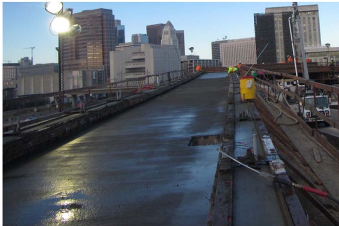
Pedestrian walkway and overcrossing poured
