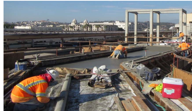
Pedestrian walkway and overcrossing poured
