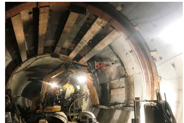
Excavation at Cross Passage 10
