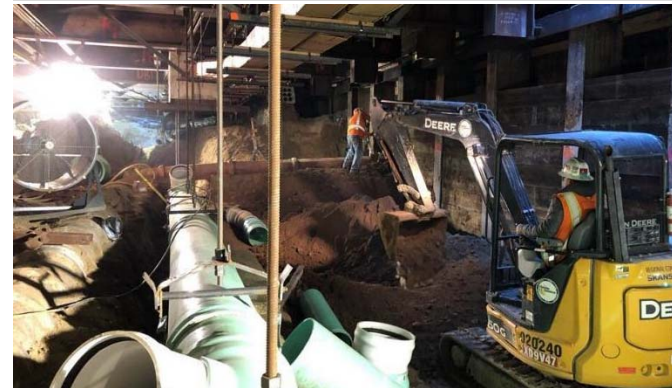
Preparations for sewer bypass under Flower Street
