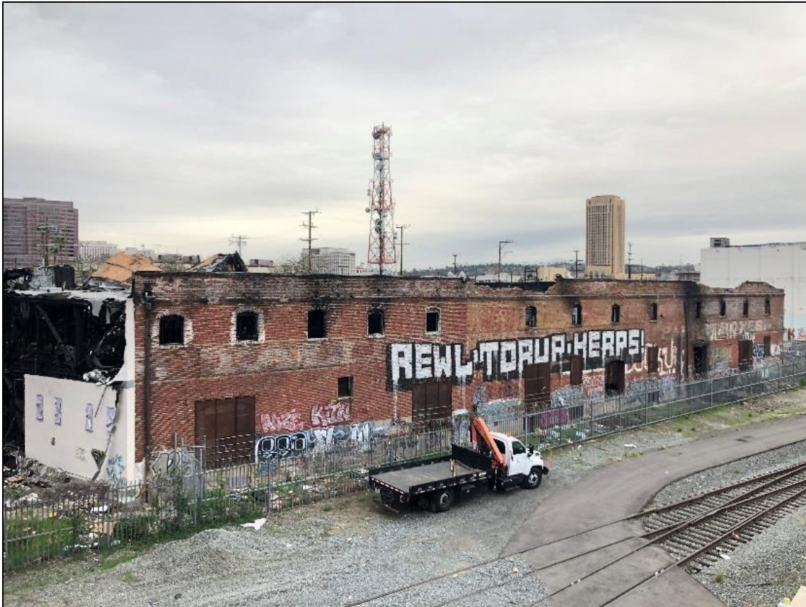
Figure 10. Citizens Warehouse/Lysle Storage Company (Pickle Works). East elevation. Looking northwest. ICF: November, 2018.
