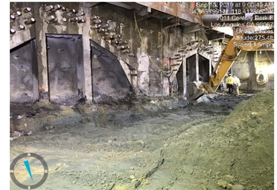
TBM Launch Box Excavation in Century City
