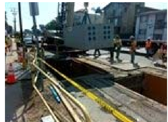
MH 500 Installation Line D
