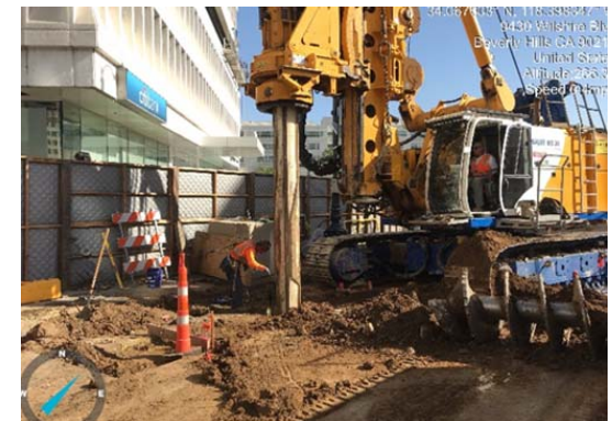
Wilshire/Rodeo Station Box Pile Installation
