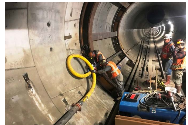
Excavation Preparation at Cross Passage 13
