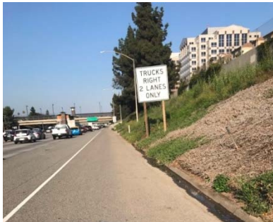
Newly Installed Caltrans Freeway Sign
