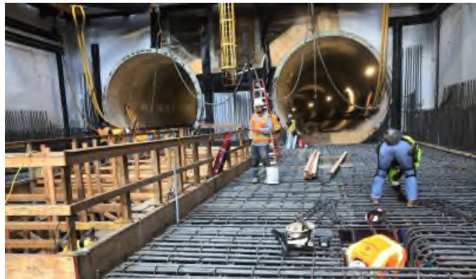
Rebar shear tie installation in Grand Av Arts/Bunker Hill Station
