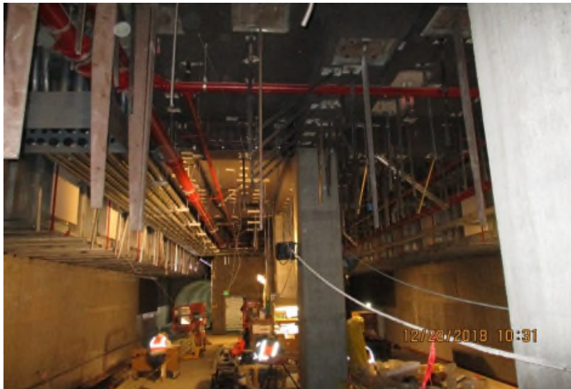
Finishes and systems installation in underground station
