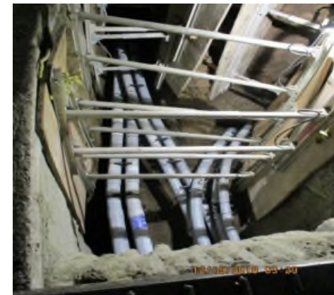
Conduit Installation on Wilshire Blvd.
