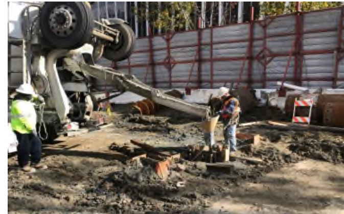
Concrete Placement at Soldier Pile in Century City
