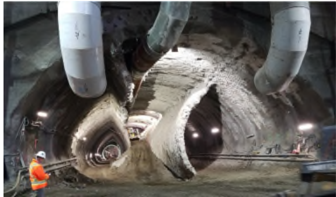
Demolition progress of central walls of SEM
