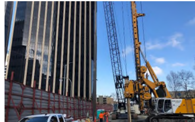
Soldier Pile Installation in Century City
